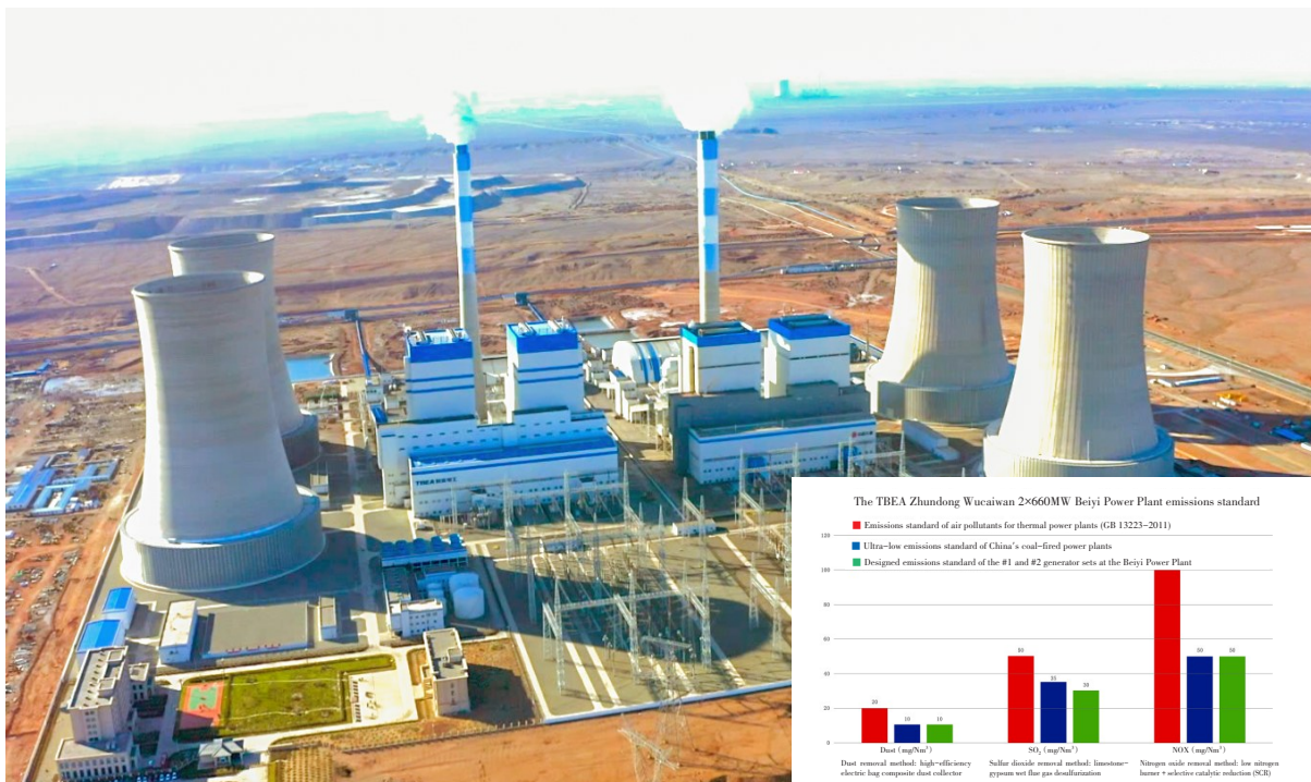
The Tianchi Energy Zhundong Wucaiwan 2x660MW Power Plant, serving China's first 1100kV UHV DC Power Transmission Project
