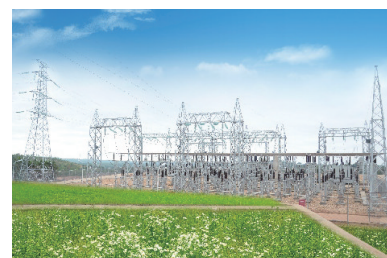
The Togo Sokode 126kV Substation and Transmission Line Project.
