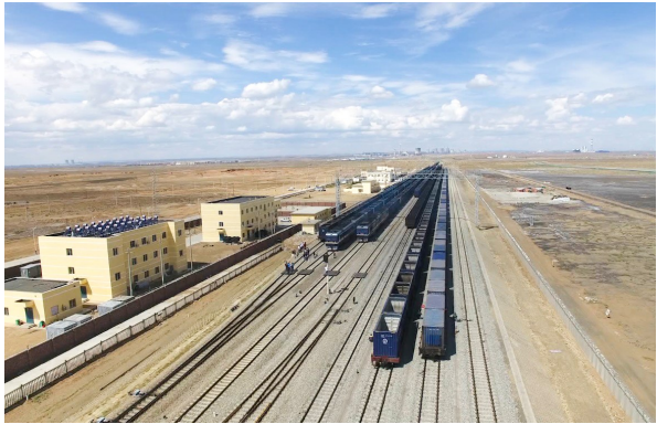
A 10,000-ton heavy haul train
