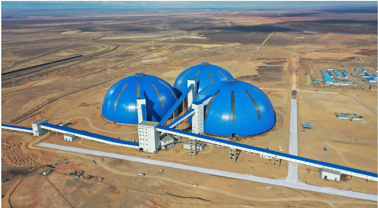
A dust control dome for coal storage yards
