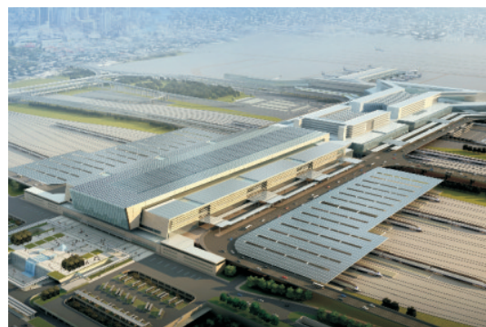
The Shanghai Hongqiao High-speed Passenger Railway Station 6.6MW Project is Asia’s largest BIPV power station.
