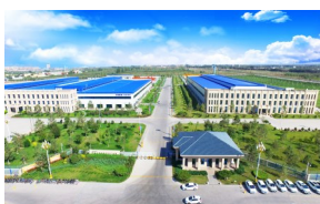
Smart Electrical Engineering Industrial Park (Changji)
