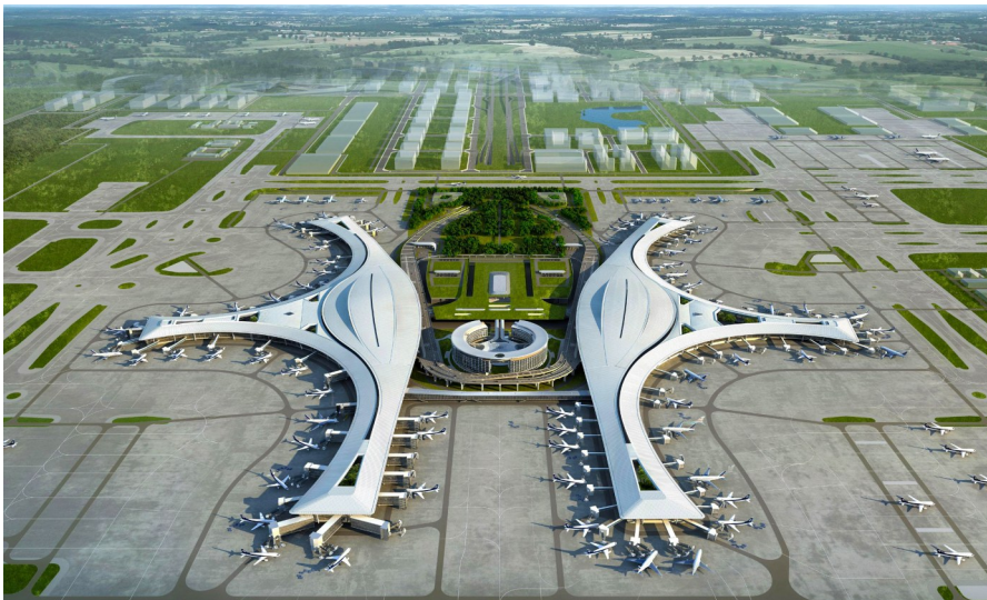
Various types of transformers, high and low voltage switchgears, pre-branch cables and other equipment are used in the Chengdu Tianfu International Airport.
