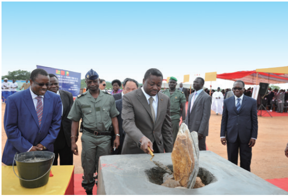
Togolese President attends the commencement ceremony of the Sokode Substation constructed by TBEA on August 30, 2013.
