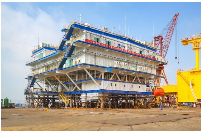
TBEA's centralized supply of primary equipment for offshore booster station successfully passes user acceptance testing and becomes the first offshore wind power supplier in China.
