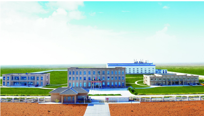
Shanshan County Dikaner Industrial Park
