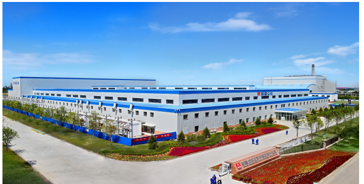
Shihezi New Material Industrial Park
