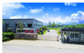
Nanjing Smart Electrical Engineering Industrial Park (Nanjing)
