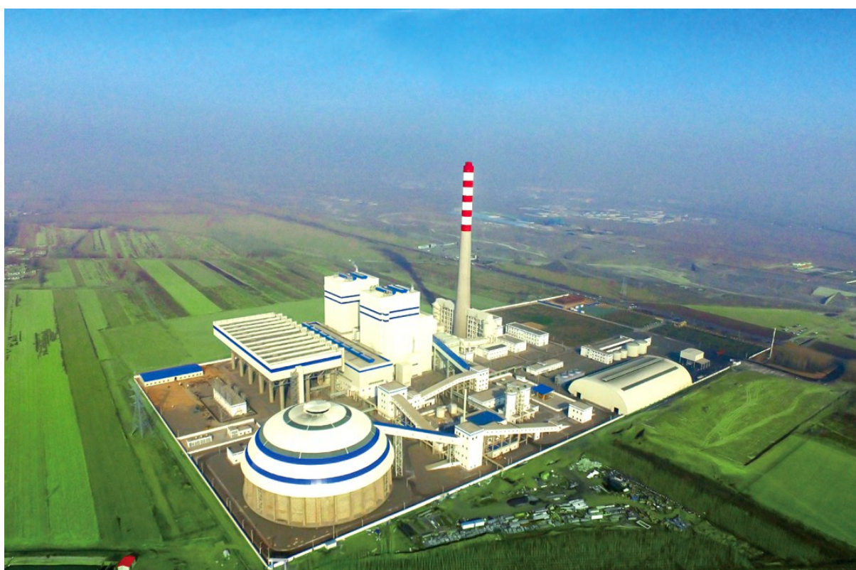
The Changji 2x350MW Combined Heat & Power Generation Project
