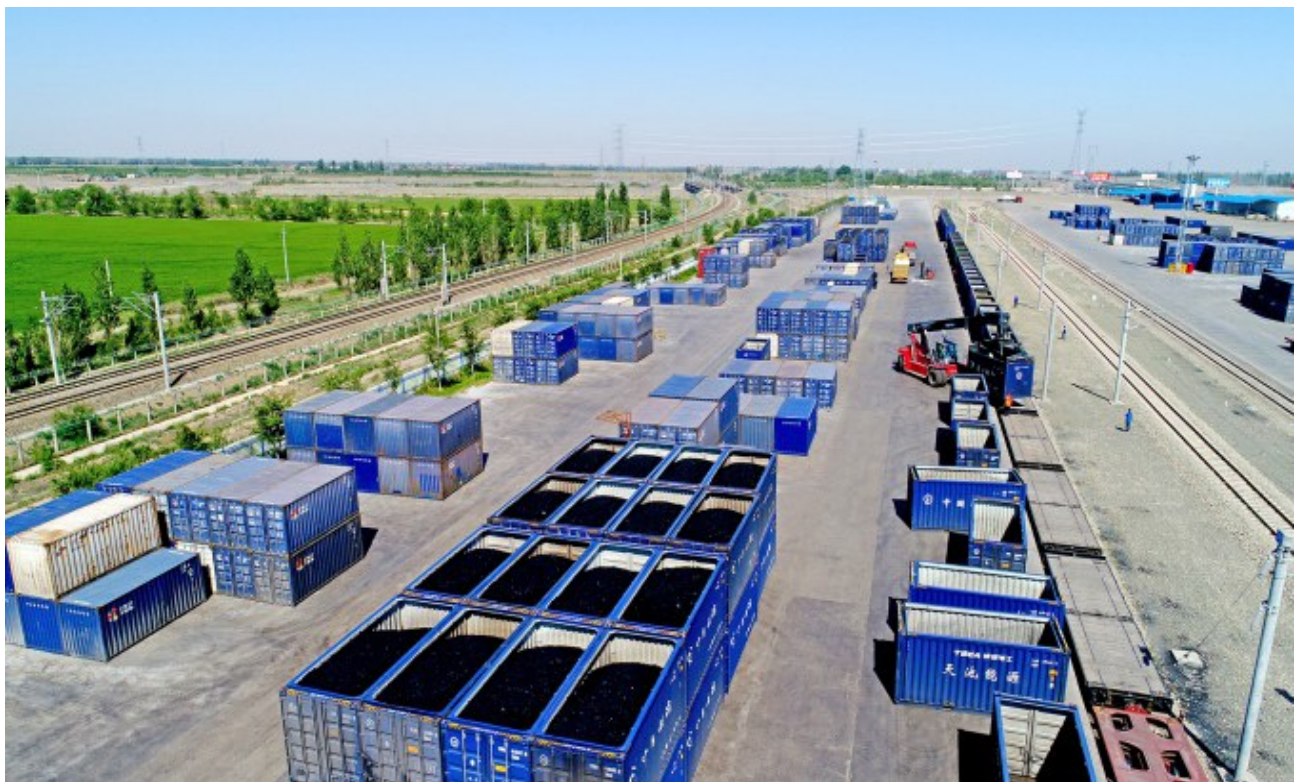
A special operation platform for Zhongjiang Logistics Co., Ltd.
