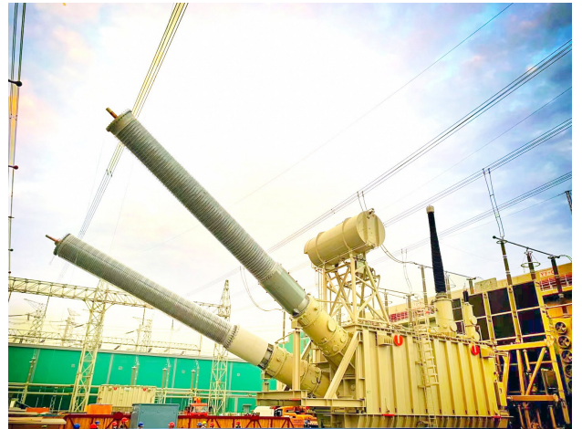
The first 800kV UHV dry-type DC bushing with independent intellectual property rights developed by TBEA is used in Qinghai-Henan 800kV UHV DC transmission project, the first UHV line designed for clean energy transmission.
