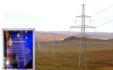
The Ulan Bator-Manderlay 330kV Power Transmission and Distribution Project in Mongolia was given the Mongolia Energy Construction Quality Engineering Award.
