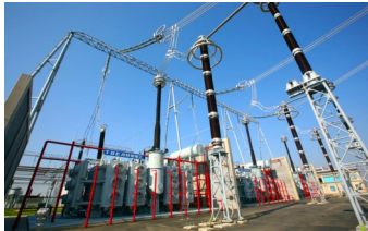
TBEA's 1000MVA/1000kV UHV AC transformer is used in the world's first commercial 1000kV Southeast Shanxi-Nanyang-Jingmen UHV Alternative Current Test Demonstration Project.
