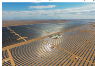
The 150MW Desert Power Station in Hami.
