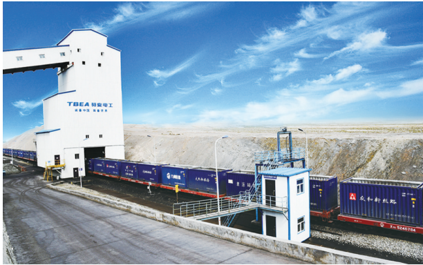
A railway automatic loading system
